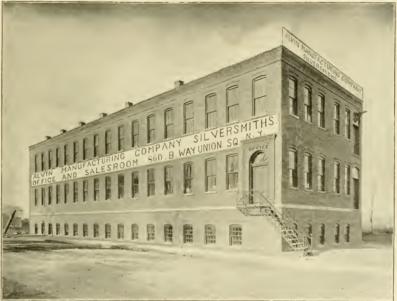
NEW PLANT OF THE ALVIN MANUFACTURING COMPANY, SILVERSMITHS, IRVINGTON, N. J.
